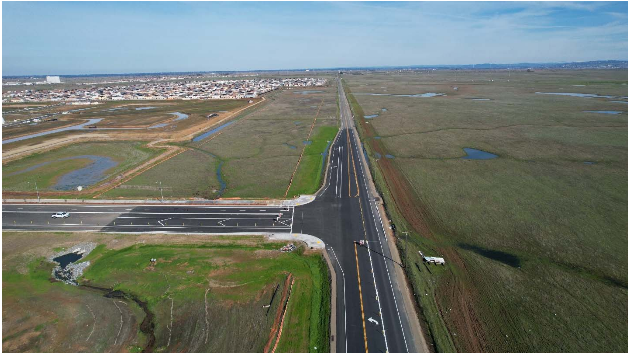
Picture 2: Along Grant Line Road, looking north
